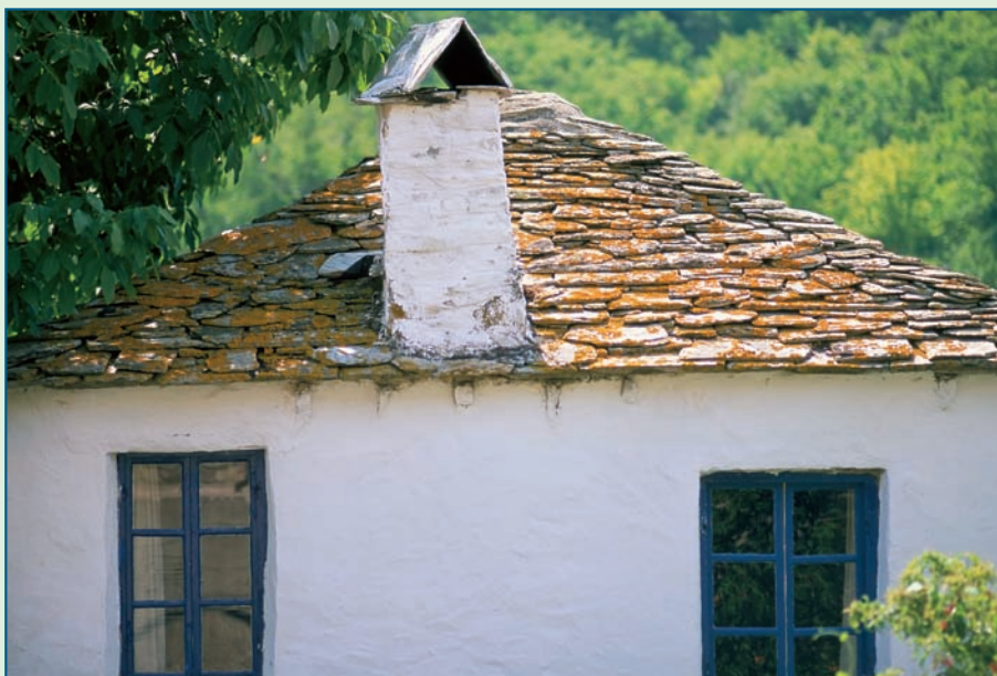
figure ar.3 This house has been painted with whitewash (a mixture of lime and water). Because lime picks up carbon dioxide from the air, it eventually turns back into chalk.
